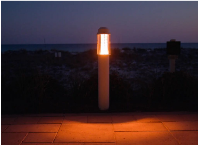
7. Long wavelength bollard light fixture. Photo: Sea Turtle Conservancy – conserveturtles.org
