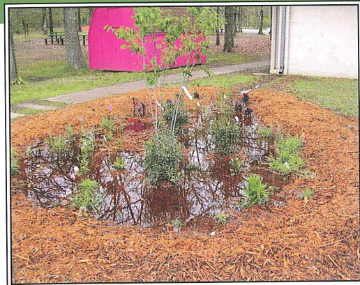
Downspouts direct roof runoff into a rain garden
