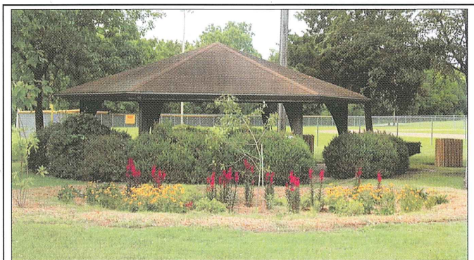
This rain garden of native trees, shrubs and perennial flowers captures stormwater runoff from a park pavilion roof
