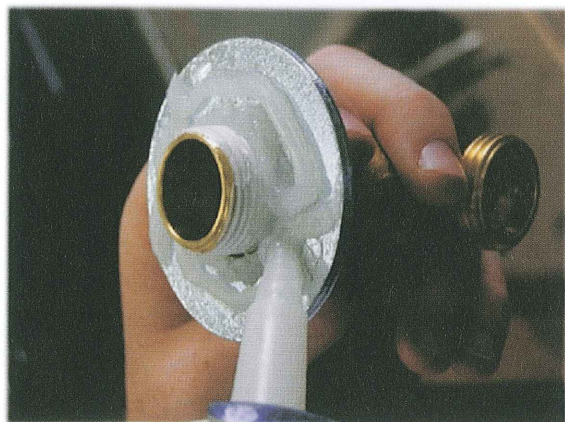
Figure 3. Teflon tape and silicone around all fittings.
