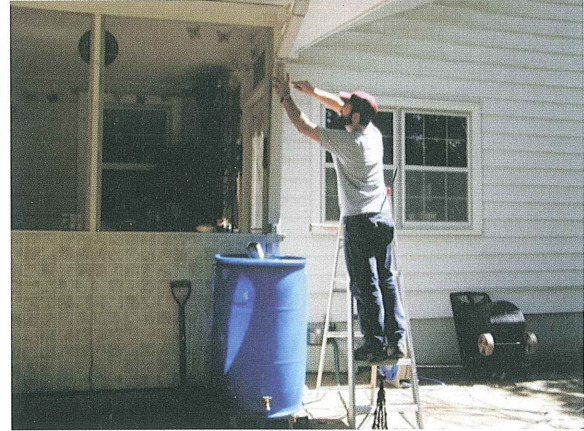
Figure 8. Re-install the downspout and connect elbow to direct water into barrel.
