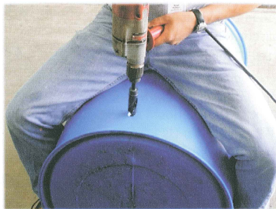
Figure 2. Drill spigot and overflow holes.
